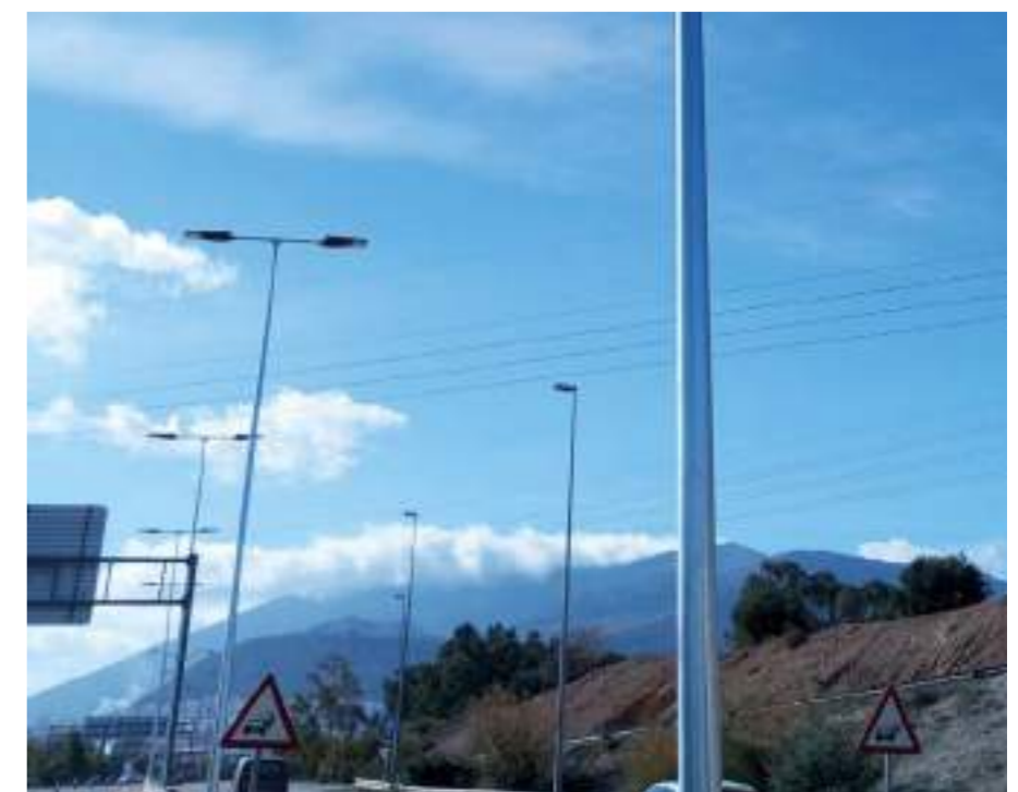
Public lighting on roads, Jaén (Spain)
