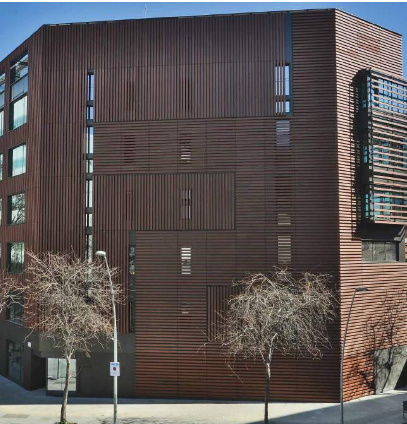
Construction and installations in Step-Up office building in Barcelona (Spain)
