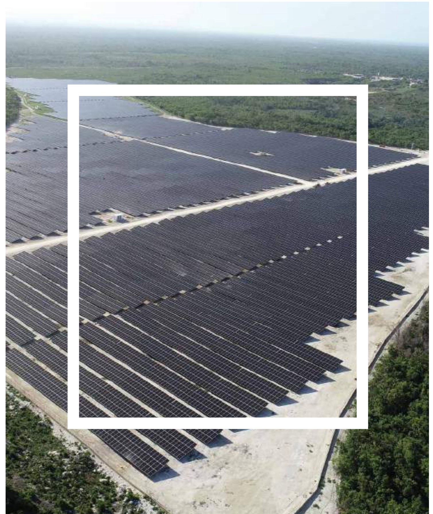
Bávaro solar photovoltaic power plant (Dominican Republic)
