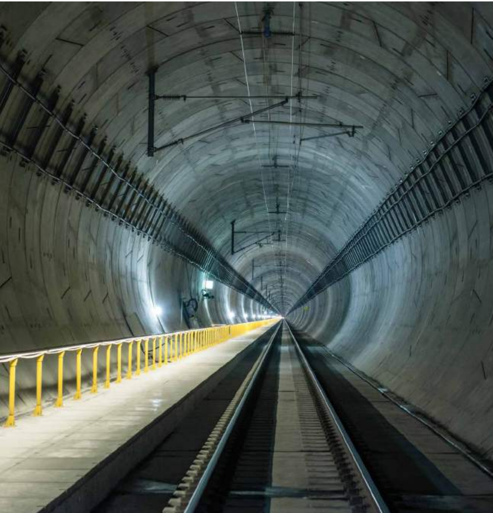
Follo Line project (Norway)
