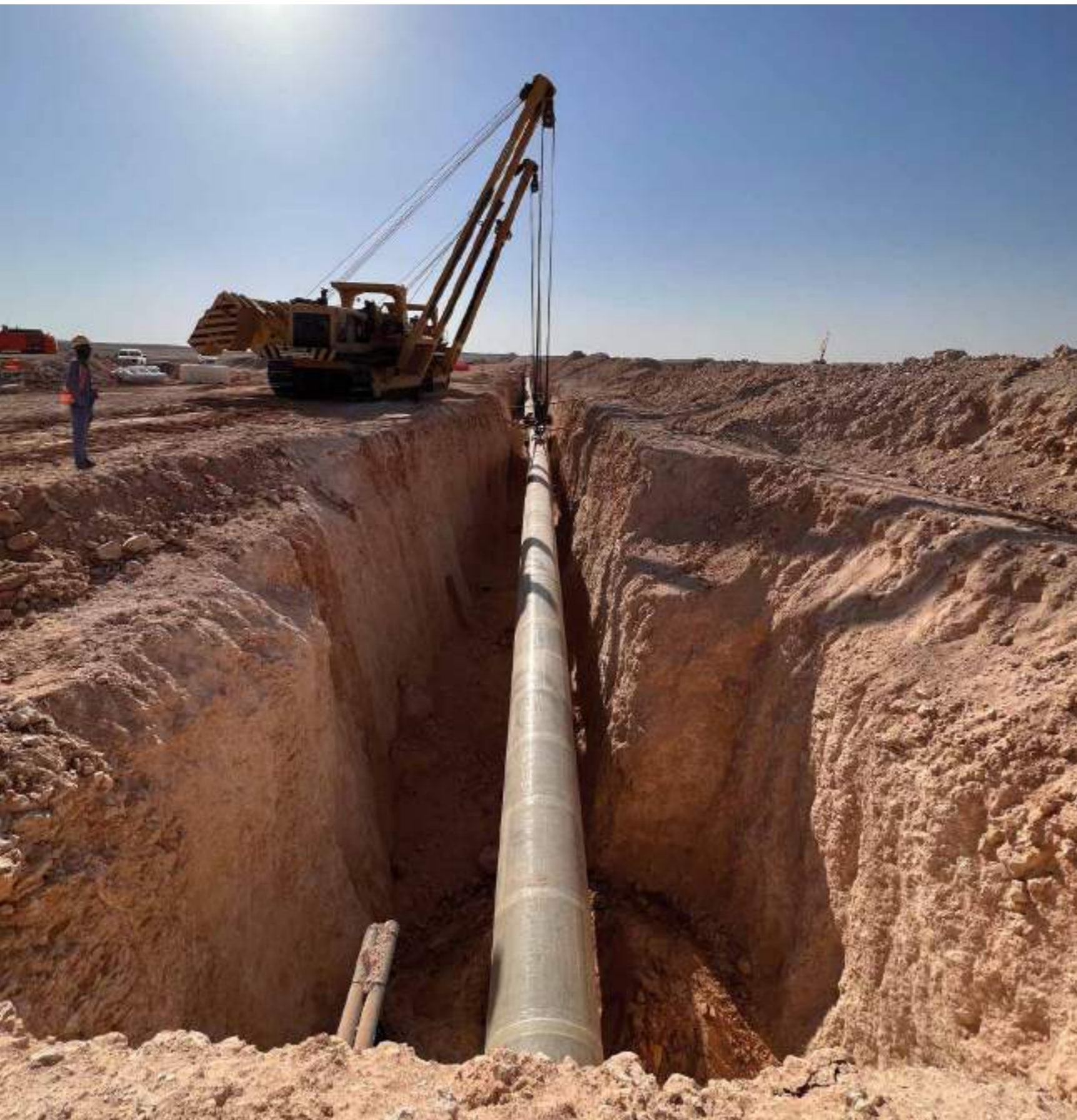
Salalah gas pipeline (Oman)
