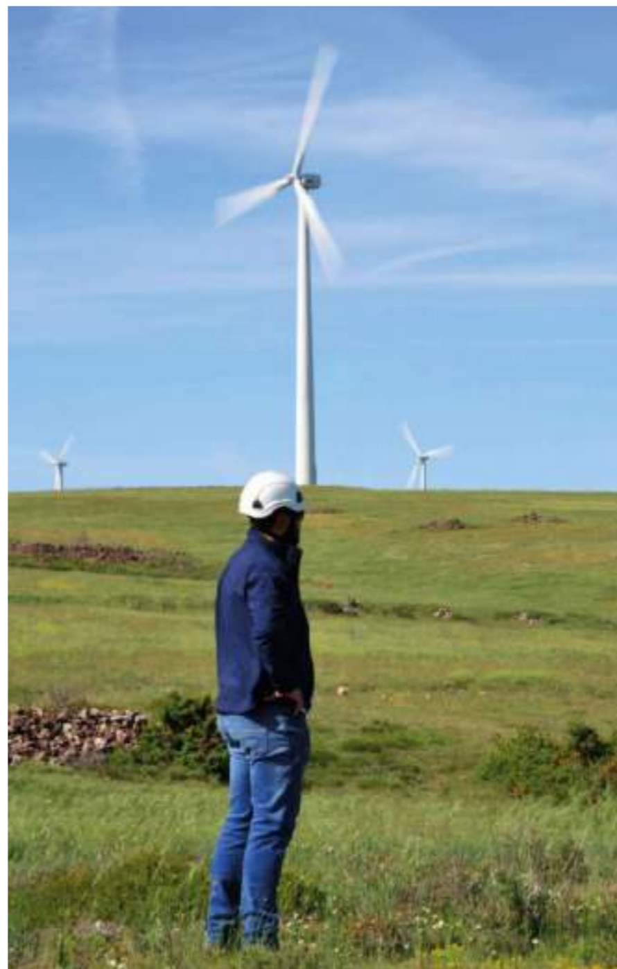
Wind farm (Spain). Enerfin
