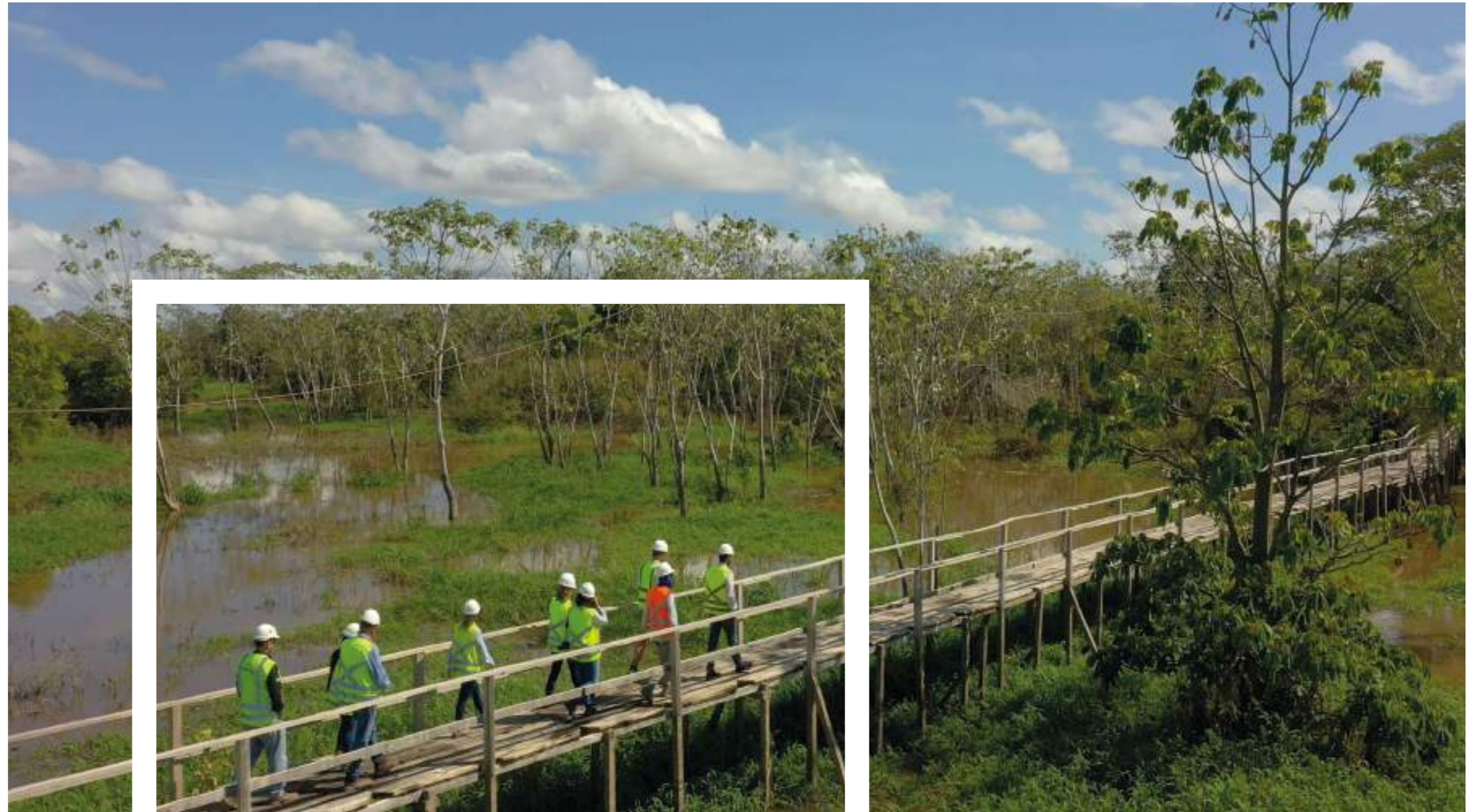
Parintins Amazonas Transmissora de Energia (PATE) line (Brazil)
