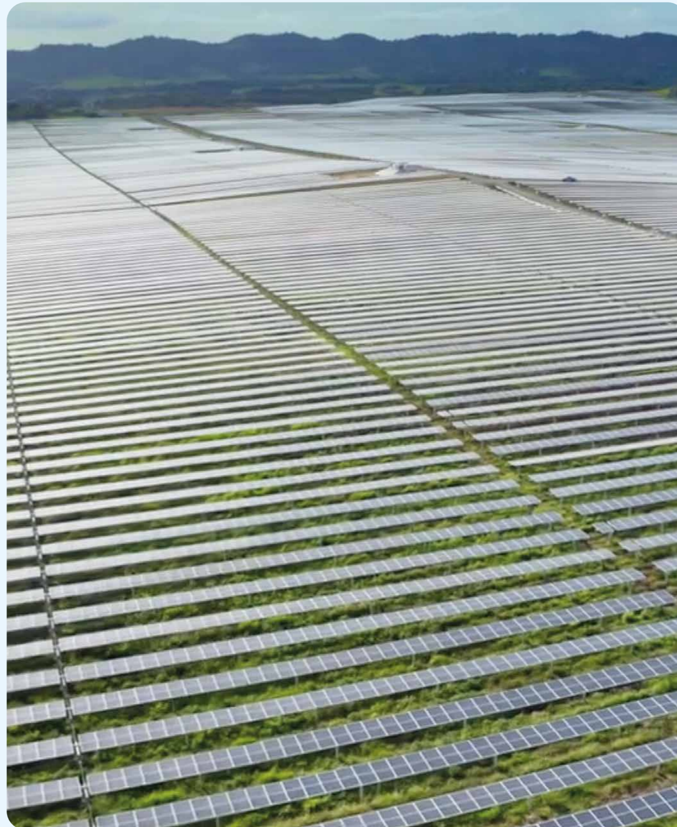
Girasol solar farm (Dominican Republic)
