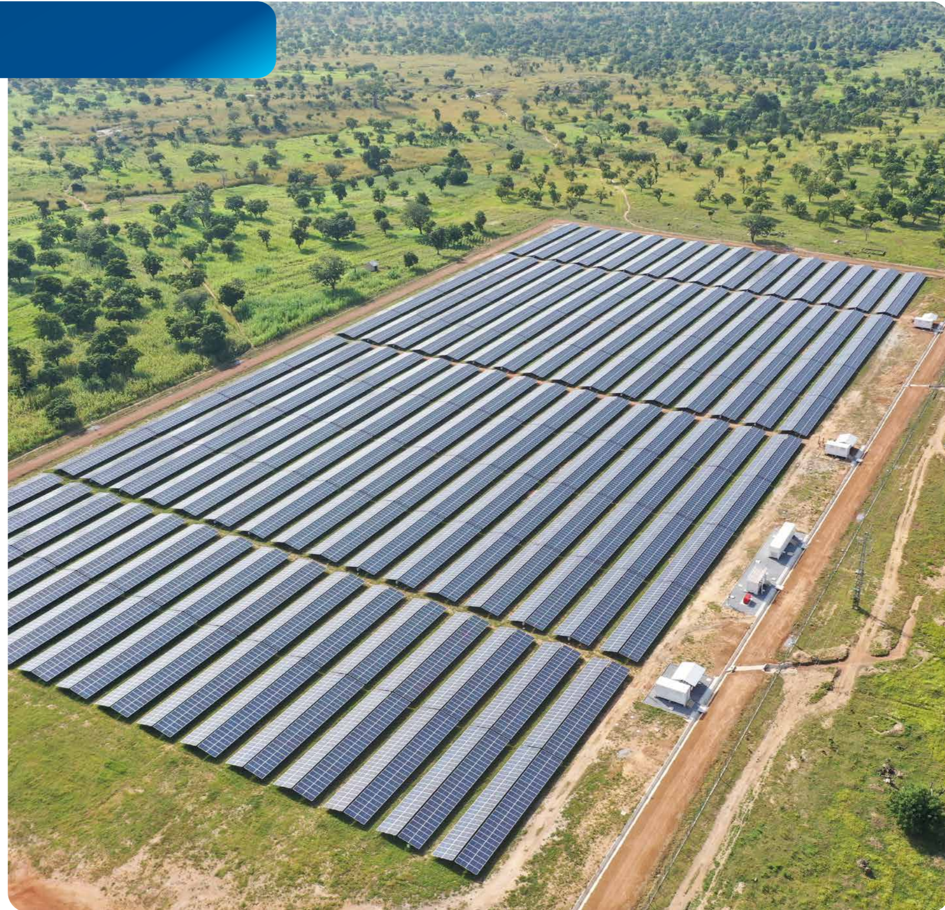
PKaleo and Lawra solar PV farm (Ghana)
