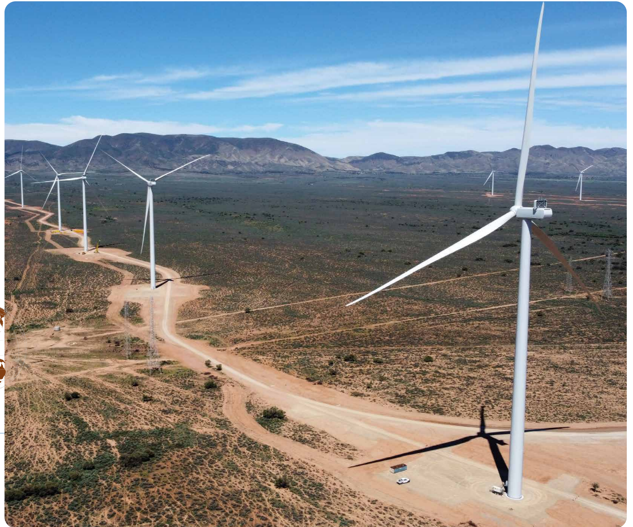
Goyder South Stage Wind Farm (Australia)
