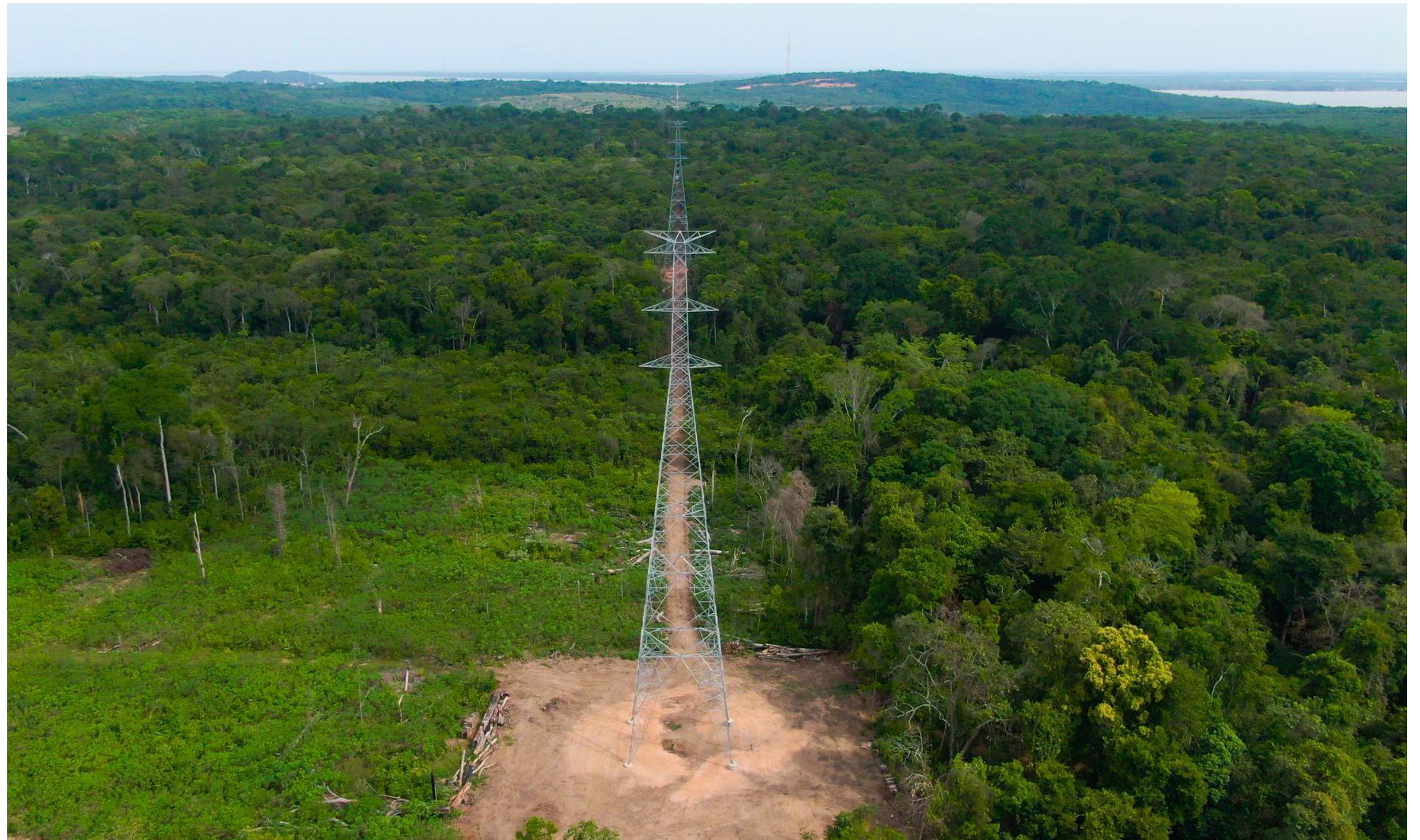
Elecnor built the tallest towers of its history, 253 meters tall (Eiffel Tower is 300 meters tall)
